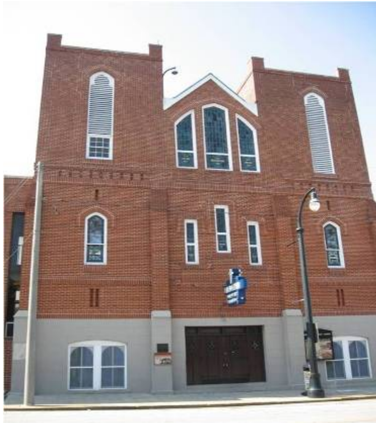
Fig. 19 – Ebenezer Baptist Church, Auburn Avenue (Atlanta, Ga).
